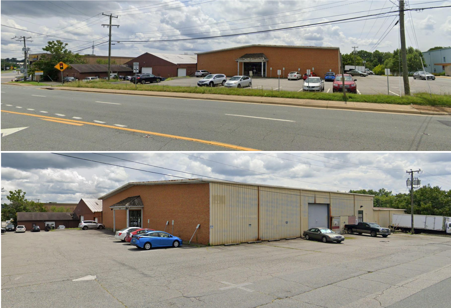
Figure 2: Views from Rio Rd. and interior to the site showing the existing conditions.
